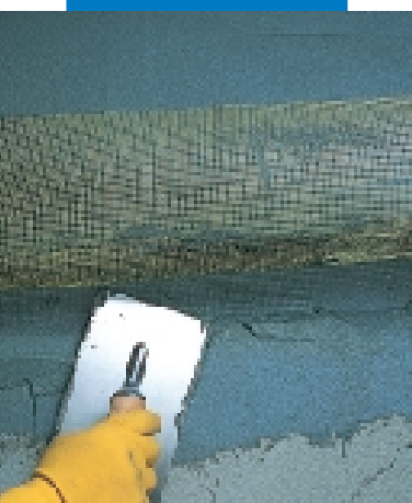
Waterproofing with Mapelastik reinforced with Fibreglass mesh
