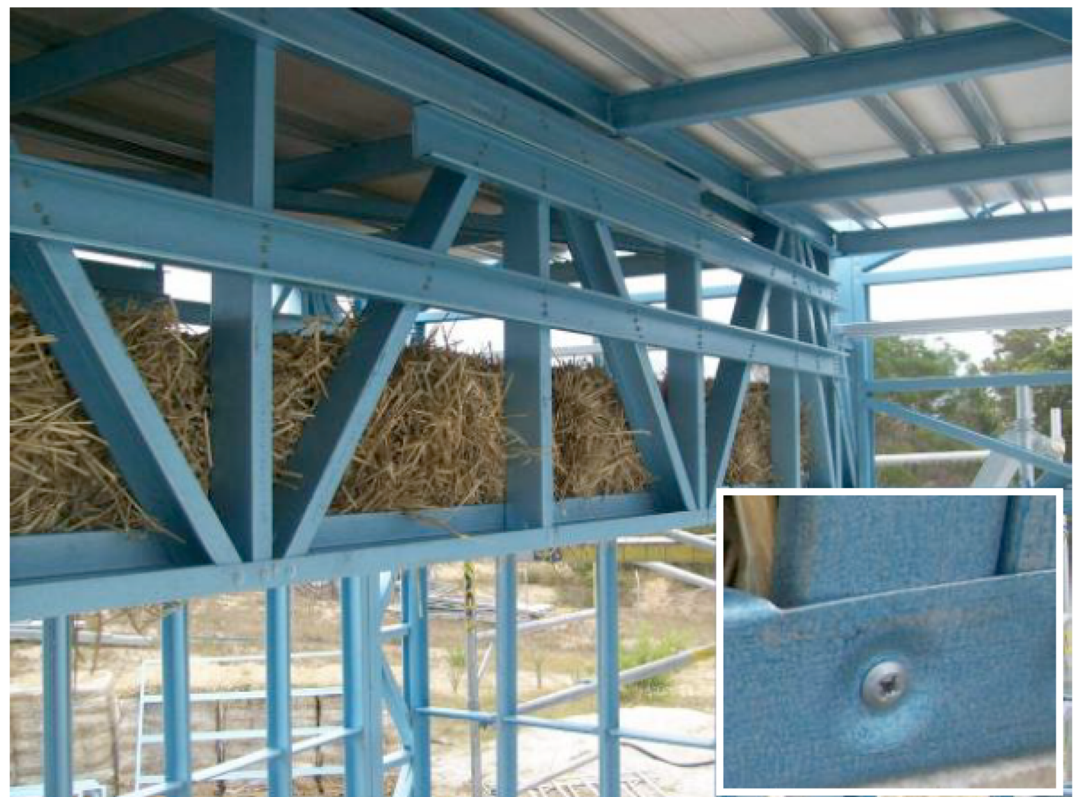
Figure 12 Light gauge steel channel sections used for framing.
